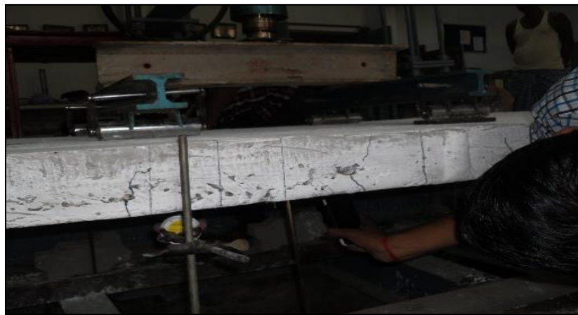
Fig. 5: Crack in Tension Zone Propagates in Upward Direction
