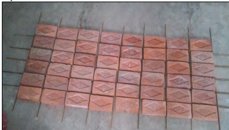
Fig. 1: Arrangement of Bricks with Reinforcement Cage
