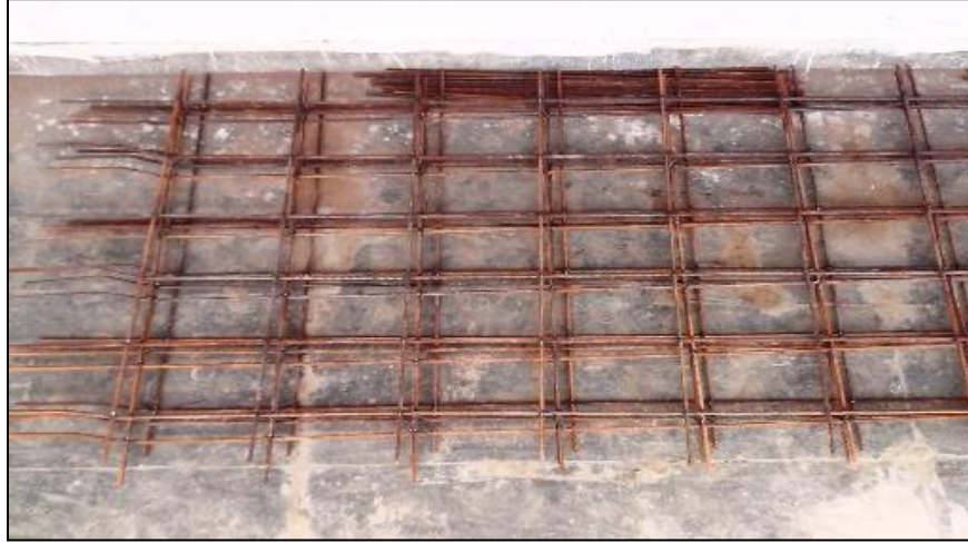
Fig. 2: Reinforcement Cage for Slabs
