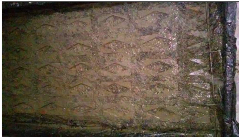
Fig. 3: Casting of Slabs
