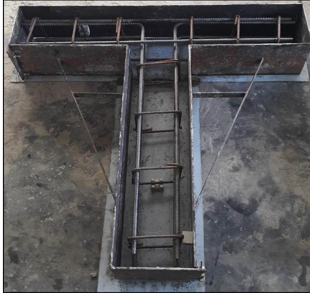
Fig. 1: Steel Mould with Reinforcement
