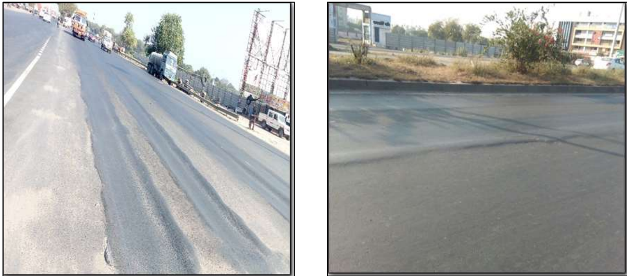
Fig. 4.4: Rutting condition
