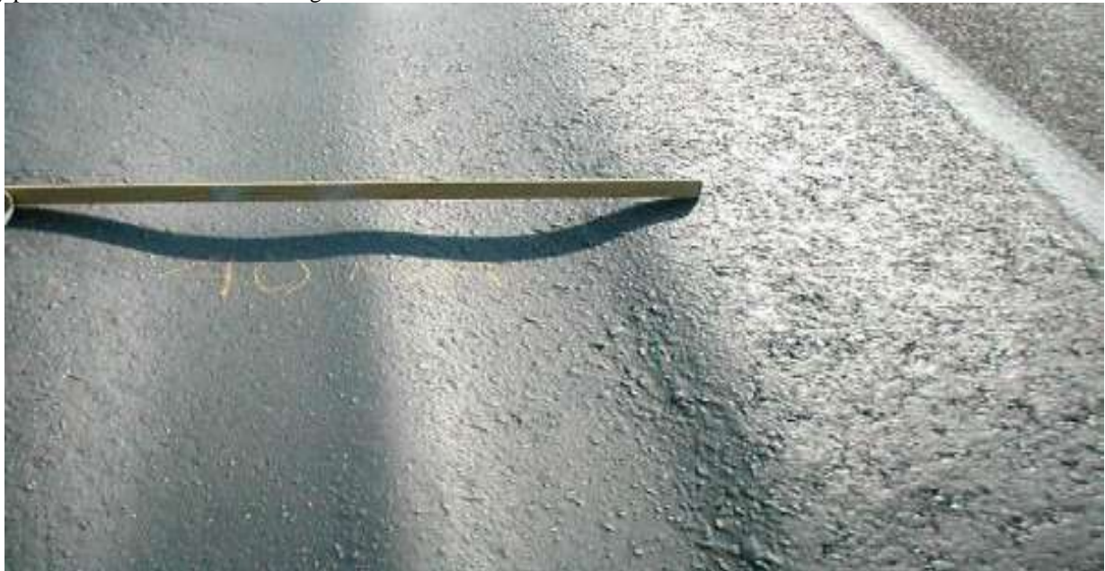
Fig. 4.3: Measurement of rutting condition
