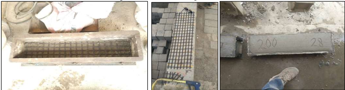
Fig. 7: Casting of Beam reinforced with Geogrid
