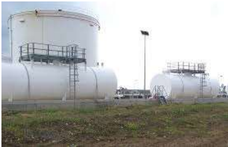
Fig. 1.3: POL Storage Tanks [3]
