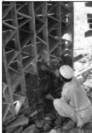
Fig. 10: Construction of Dhajji wall with stone and mud mortar inside diagonal bracing
