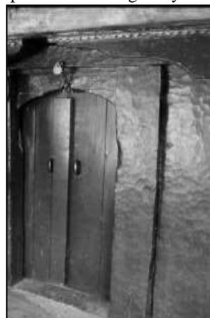
Fig. 7: Small reinforced openings are key features of Kat-Ki-Kuni.(This beautifully hand-crafted door in the maharaja of Kullu's palace has elements hewn from solid blocks of wood. )
