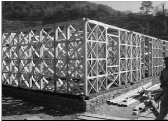
Fig. 9: Dhajji frame under construction
