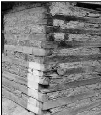
Fig. 4: Corner construction detail of Kath-Ki-Kuni style housing. (The timber bands run along both sides of the wall and are connected by pins along their length and at the corners)
