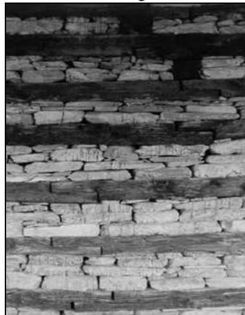
Fig. 6: Detail of Dressed stone in Kath-Ki-Kuni structure. (The use of long, flat stone distributes the compressive loads evenly)
