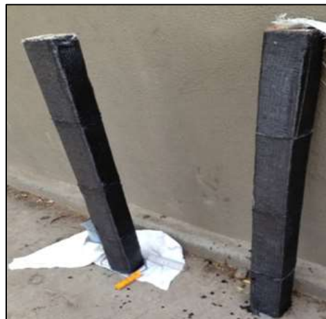
CF for Axial Beams in Construction
