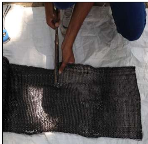
Cutting of Carbon fabric
