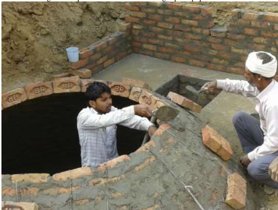
Fig. 4: Construction of Deenbandhu biogas plant
